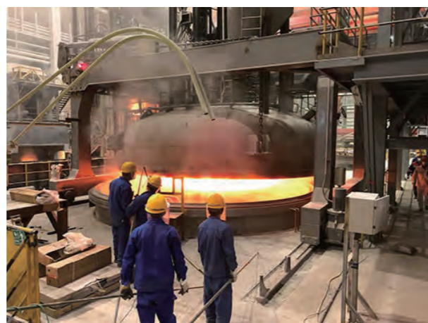
150t VOD Vacuum Refining Furnace
