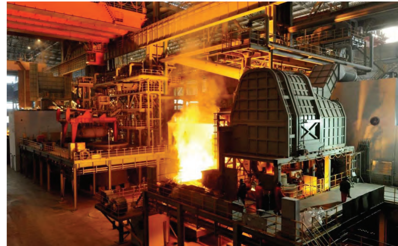
200t Ladle Furnace
