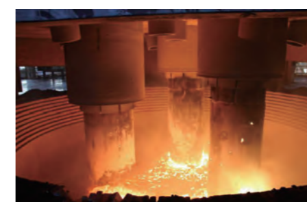
30000kVA FeSi Submerged Arc Furnace
