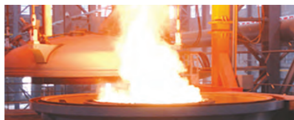
80t VD Vacuum Refining Furnace
